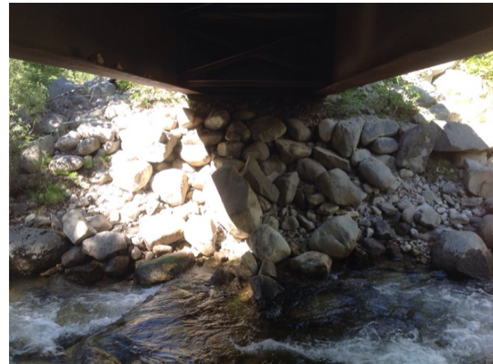
Right Bank Abutment when facing downstream
