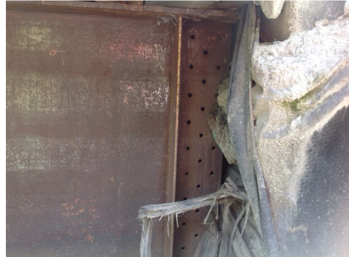
steel girders only a section of planned spliced girder
