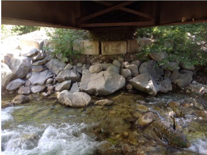
Left Bank Abutment when facing downstream
